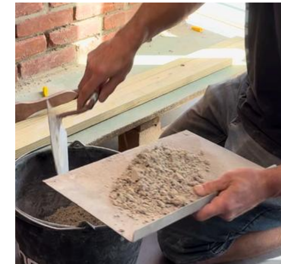
1 Take the mortar on the plate
